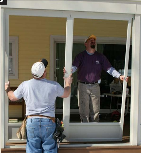
Slide the pair of wall panels up into the deeper top track until they clear the bottom of the opening, then drop the panels into the base track.
