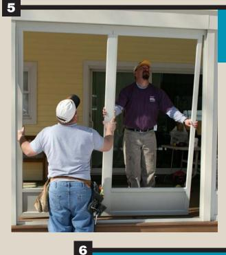
Adjust both panels to fit evenly and securely in the H-channel and the F-channels. Slide the pair of wall panels up into the deeper top track until they clear the bottom of the opening, then drop the panels into the base track.
