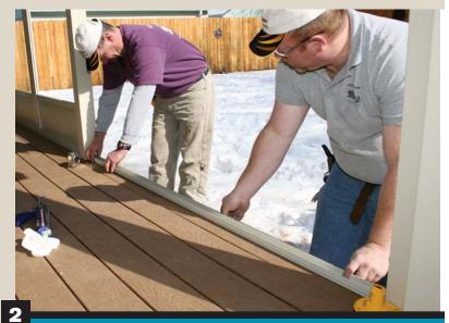
Bed the base track in caulk and screw it to the decking. Attach the top track, which is deeper than the bottom one, the same way. Drill weep holes in the base track 3 inches from the ends and 16 inches on-center.
